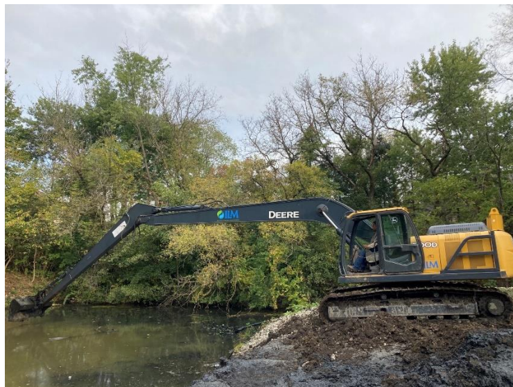
Mechanical Dredging Operation (photo source: ILM Environments)
