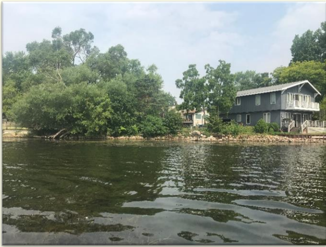
Photo #3: Example of aging rip-rap installation.
