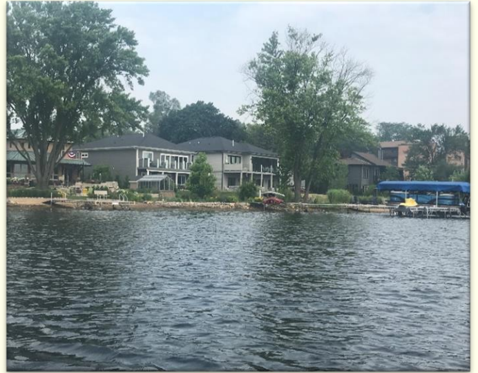
Photo #10: More areas with aging shoreline control techniques. Often experiencing moderate erosion. Landscape species near the shore should be appropriate natives to enhance erosion control.
