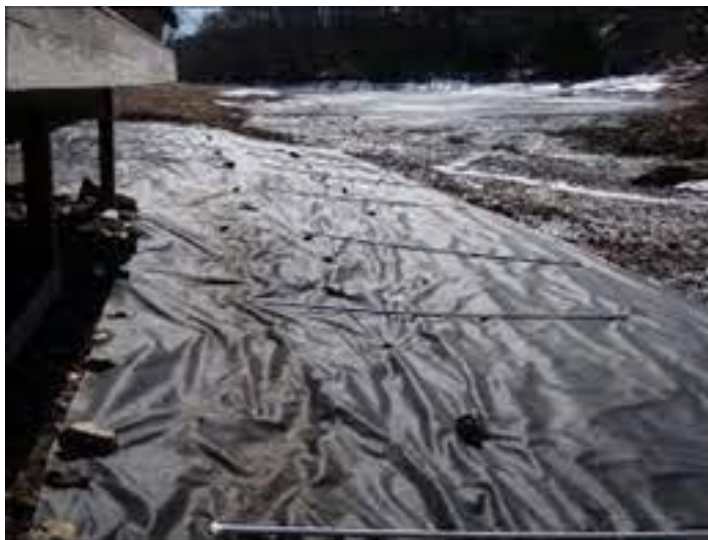
Weighted sheet mat (photo source: Wayne County, NY Soil and Water Conservation District)
